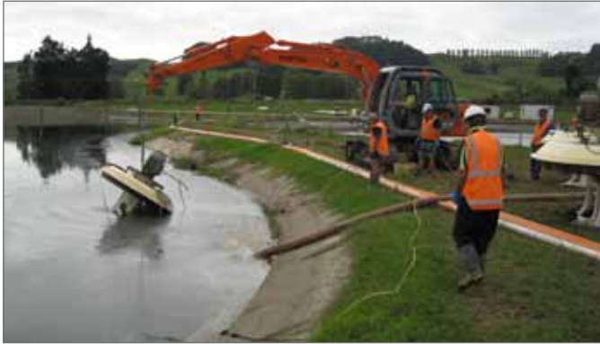
TE KUITI WASTEWATER TREATMENT PLANT UPGRADE
